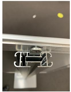
Continue to slide in the frame downwards. Make sure the top attachment goes into the channel as well.
